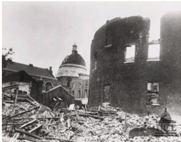
Wartime bomb damage to UCL, viewed from the south east.
